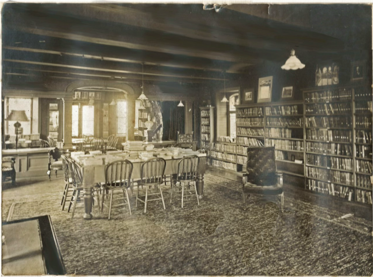
Interior of Essex Free Library, circa 1905. The area of the library in the far background, beyond the arches, is now known as the Dorothy B. Voorhis Reading Room. Archival photograph, Belden Noble Memorial Library.
